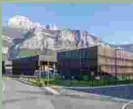
CENTRE TECHNIQUE MUNICIPAL Crolles
